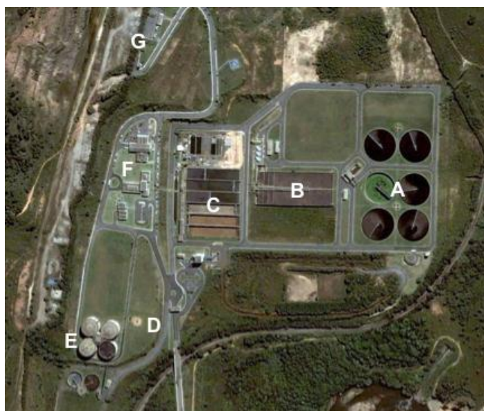
Figure 1. Aerial view of ETE Arrudas (Date of the image: 12/05/2007). A) Main entrance B) Control and support facilities C) Anaerobic digesters D) Biogas flares E) Primary decanters F) Aerobic reactors G) Secondary decanters.
